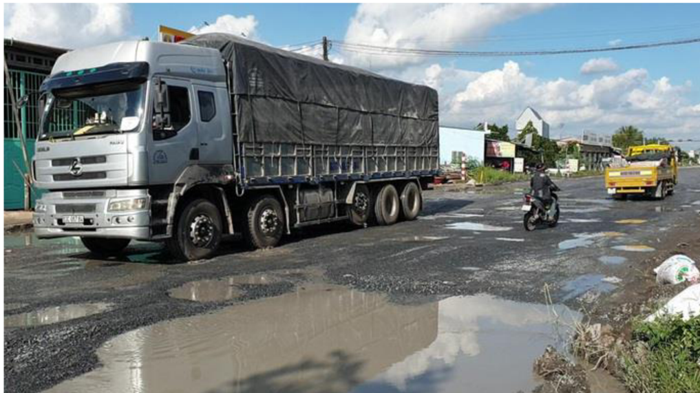
Image 2. Cai Lay bypass road (Tien Giang province) is seriously degraded
