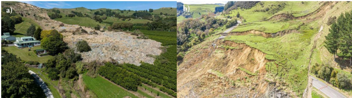
Figure 2. Examples of landslides in New Zealand: a) Manutuke landslide triggered by cyclone Gabrielle, 2023; b) Whanganui landslide destroyed the state highway, 2019 (Images taken from Dave Petley’s blog).
