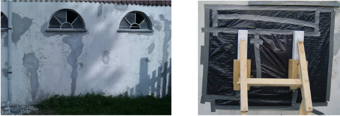
Fig. 7 The reference old stable for the pilot test.
