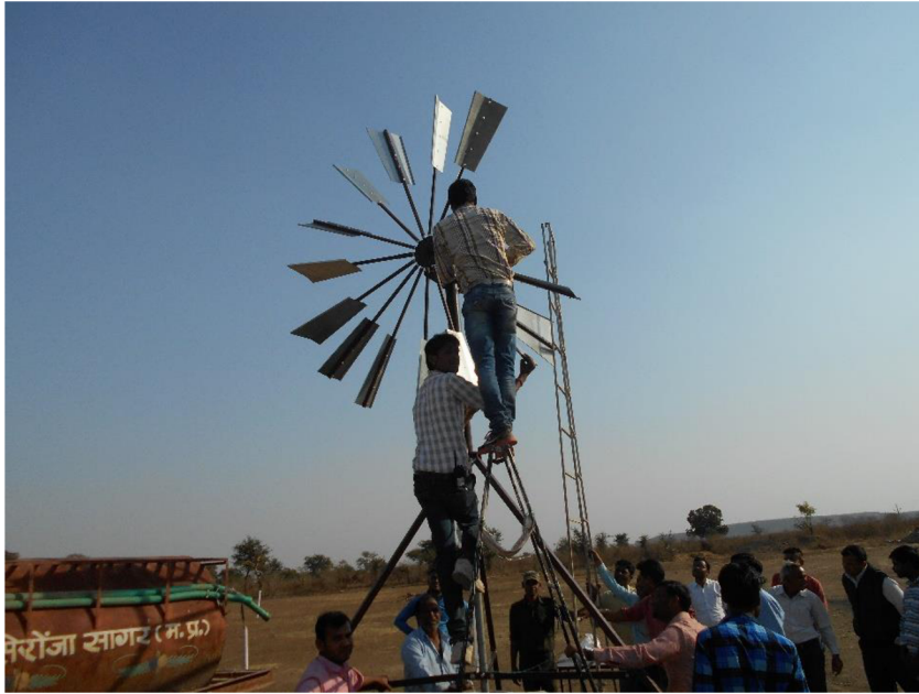
Figure 18 Wind pump construction in India
