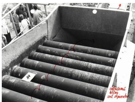
Obr. 43 – Odlučovač hlíny (Modřany) [46]
