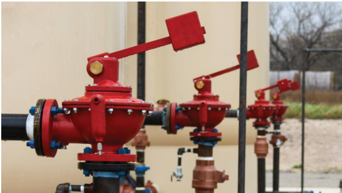
Figure 6: Control Valves for Two-Phase Separation (Fadaei et al, 2021)
