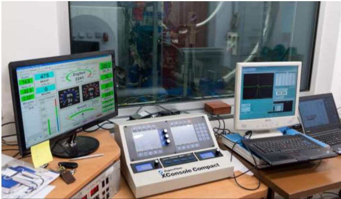
Figure D.1 Engine test cell control room
