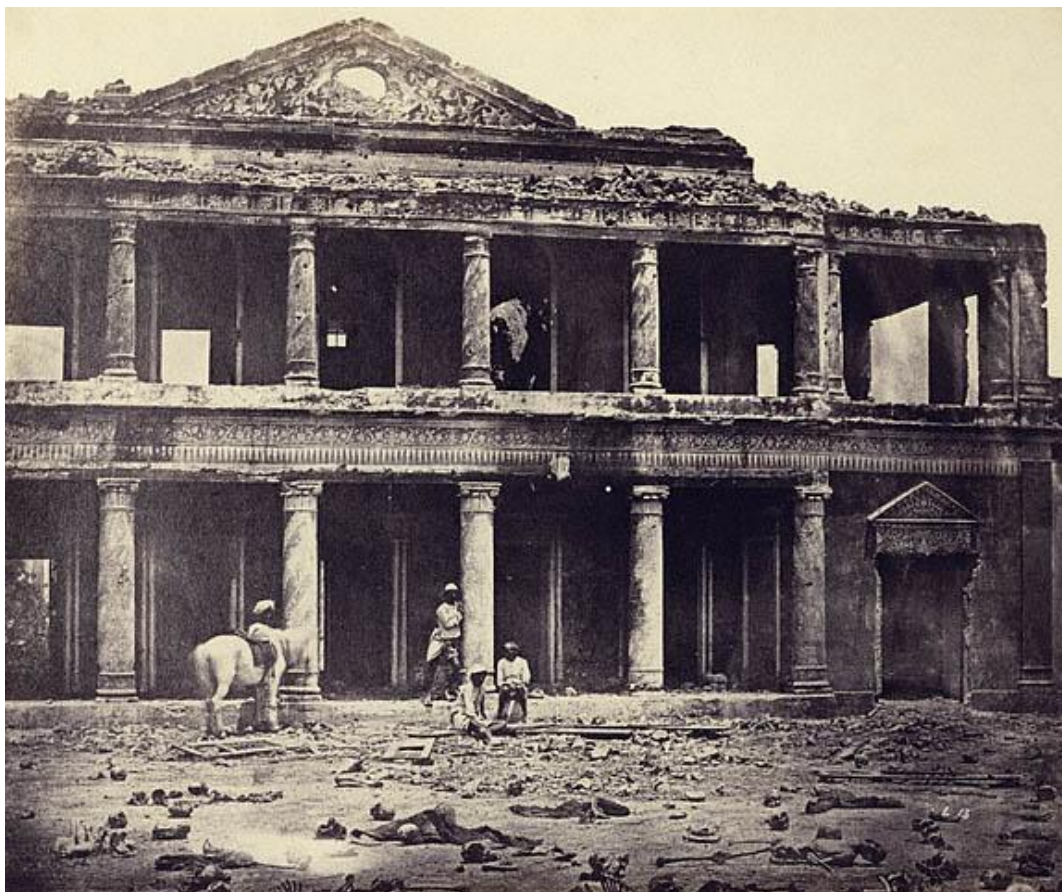
Obr. 3.: Interior of the Sikandar Bagh – Felice Beato, 1858
