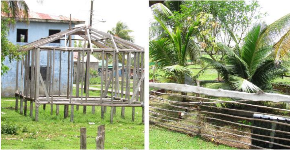
Fig. 4 Mangrove used as a construction material in the local community
