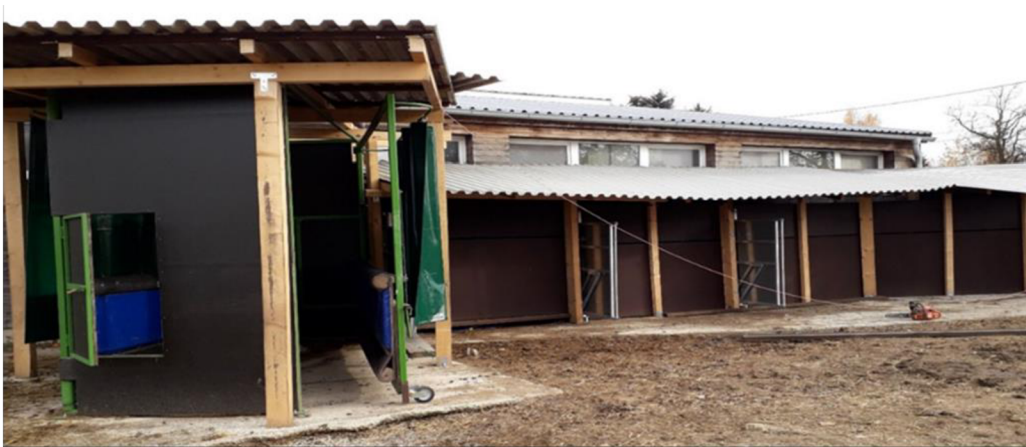
Figure SM5.1. A side view picture of the raceway and squeeze chute handling system, showing the galvanized sliding doors, the green plastic curtain, and the blue coloured adjustable padded boards on the rotating doors.
