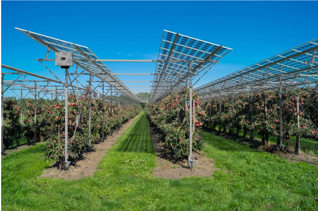
Figure 13: Overhead solar system, Austria, Heidegg (ecowind.at, 2023)
