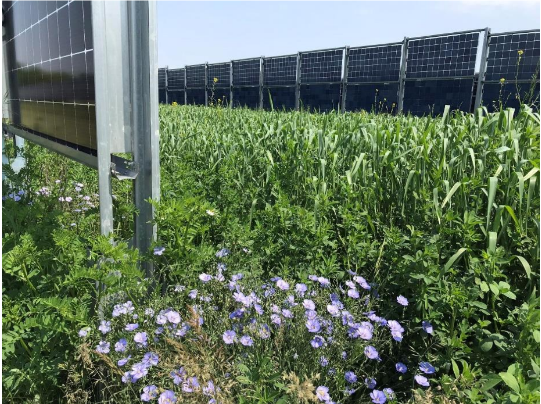
Figure 9: Experimental interspace agrivoltaic system in Austria, University of Natural Resources and Life Sciences, Vienna (Pechlátová, 2023)
