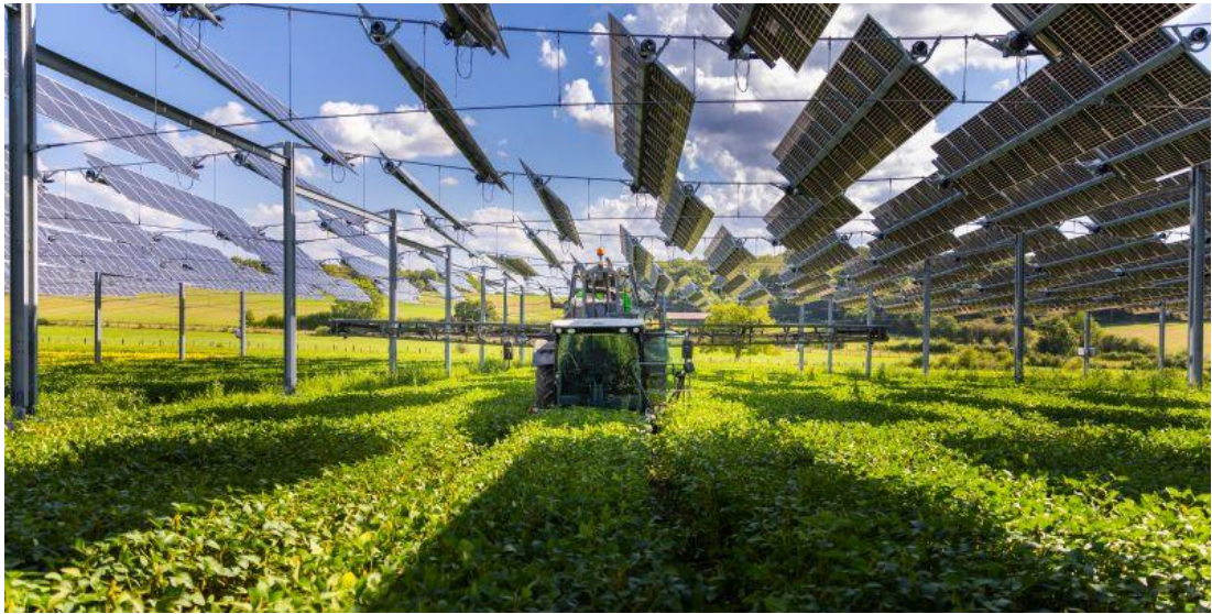
Figure 12: Elevated agrivoltaic system, France (Tse.energy, 2022)
