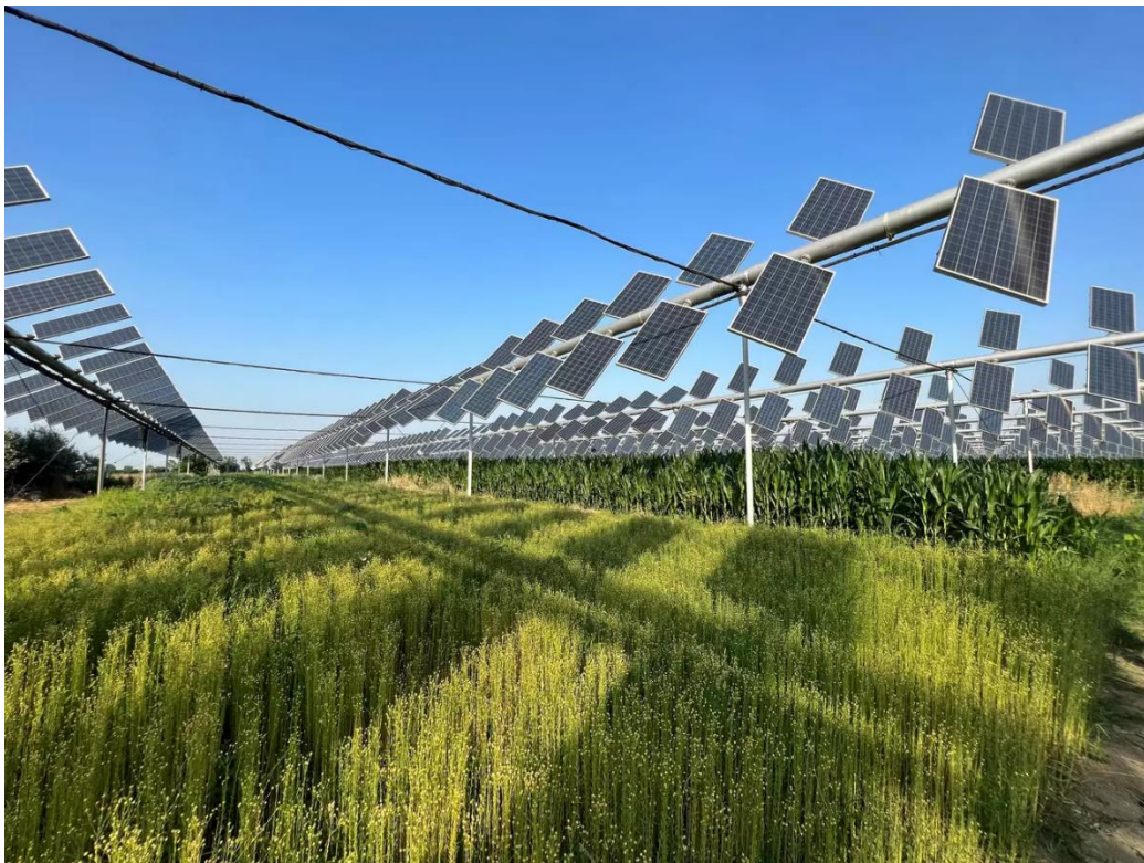
Figure 16: Stilted agrivoltaic (Bim & Neugebauer, 2023)
