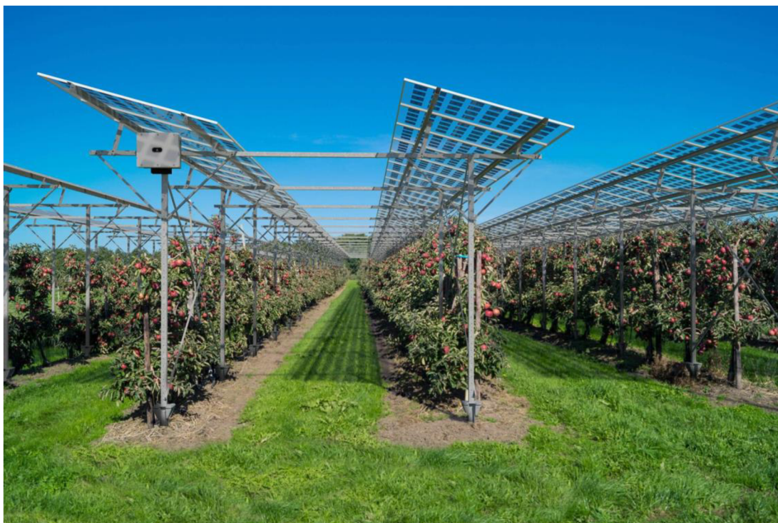
Figure 13: Overhead solar system, Austria, Heidegg (ecowind.at, 2023)
