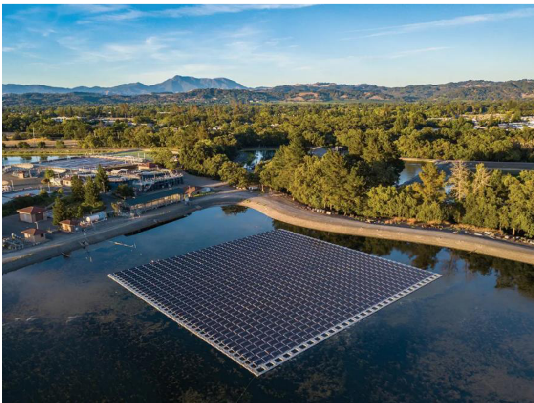
Figure 19: “Floatovoltaic” in Windsor, CA - “solar pond” (Collins Electrical Company INC, n.d.)
