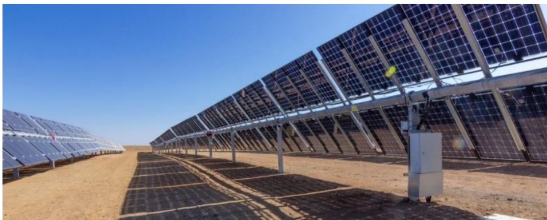
Figure 7: Bifacial solar panel - generating electricity on both the front and back of the solar panel (DNV, 2022)
