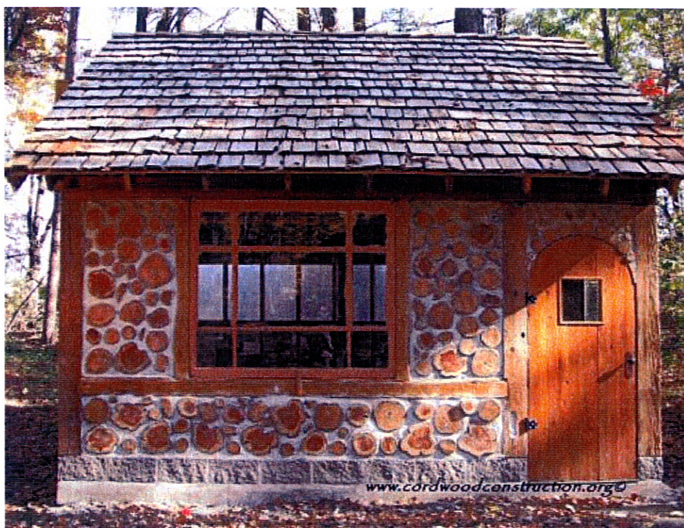
Obr. 4: Vzor stavební technologie „cordwood“ (zdroj: https://cordwoodconstruction.wordpress.com/2017/05/16/cordwood-cottage-garden-shed-recycled/ )
