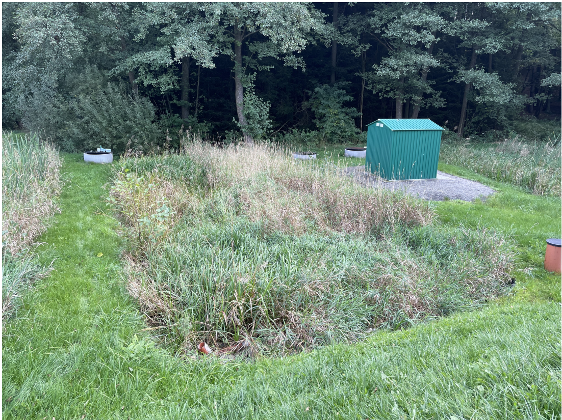
FIGURE 4.2: Experimental constructed wetland M2 with horizontal subsurface flow near Veliký Rybník (Vymazal, September 2021).
