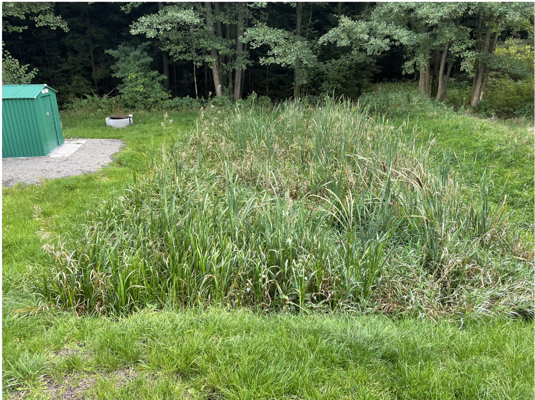
FIGURE 4.3: Experimental constructed wetland M3 with horizontal subsurface flow near Veliký Rybník (Vymazal, September 2021).
