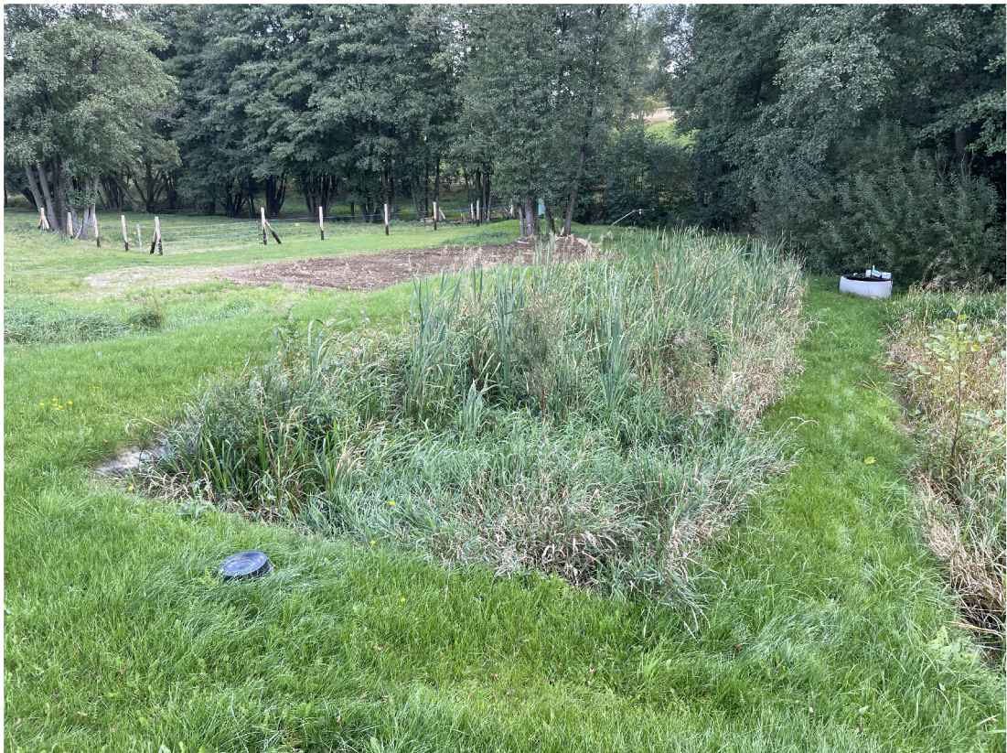
FIGURE 4.1: Experimental constructed wetland M1 with horizontal subsurface flow near Veliký Rybník (Vymazal, September 2021).
