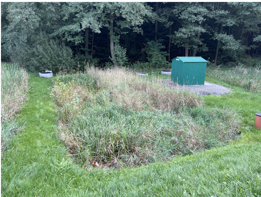
FIGURE 4.2: Experimental constructed wetland M2 with horizontal subsurface flow near Veliký Rybník (Vymazal, September 2021).
