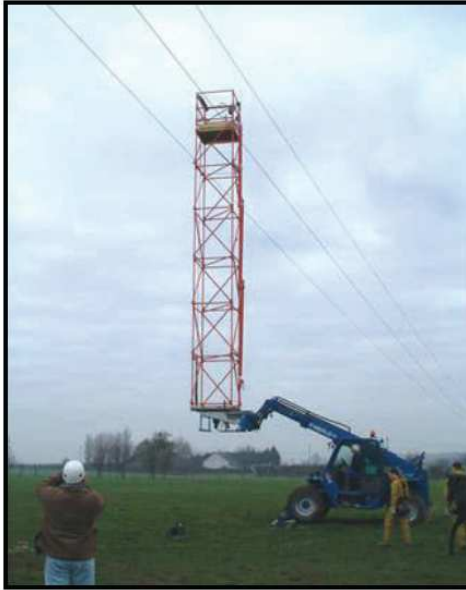
Figure 2-3 Live-line installation [1]
