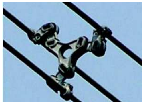
Figure 3-15 Triple spacer-damper with two articulations per arm and hinge type clamps [2]
