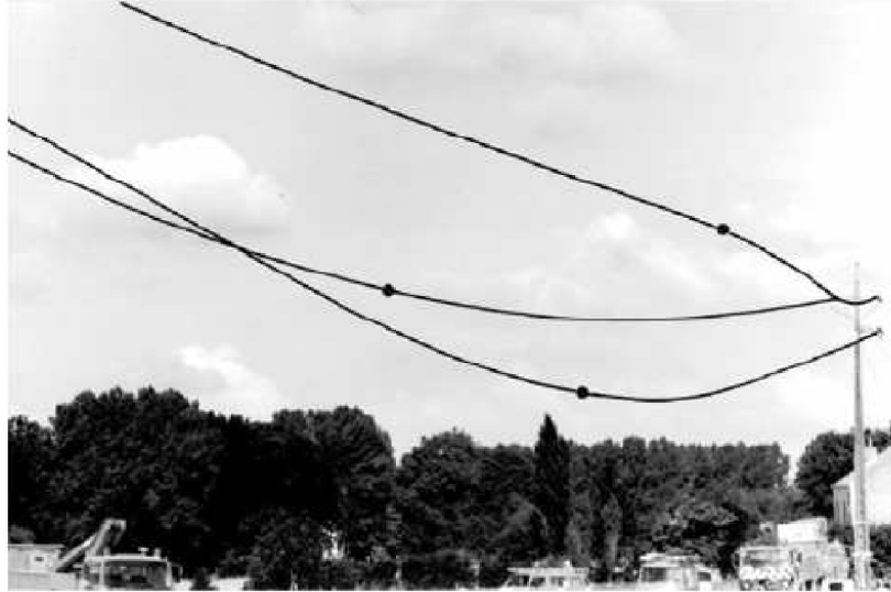
Figure 3-19 Instantaneous position of the conductors taken during three-phase short-circuit test on 15-kV [2]
