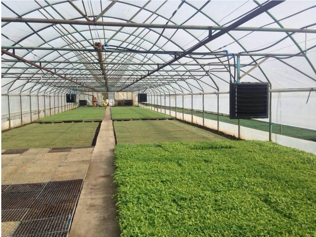
Picture 4: Quonset greenhouse
