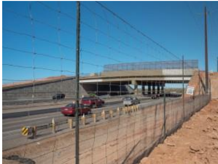
Figure 7. Road fencing (photo by Thomas Wiewandt).
