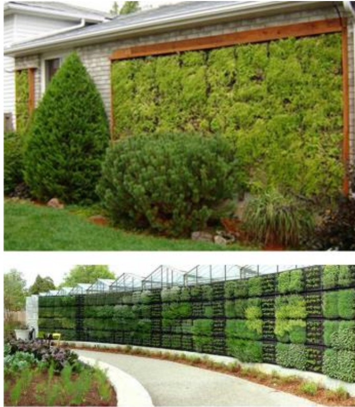
Figure 9. Modular Living Wall Canada (above), Atlanta Botanical Garden (below). Source: (Burhan & Karac, 2013)
