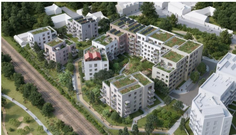
Picture 11: Visualization of the residential area showing green roofs, solar panels, green infiltration surfaces and many public green areas (Skanska, 2021).
