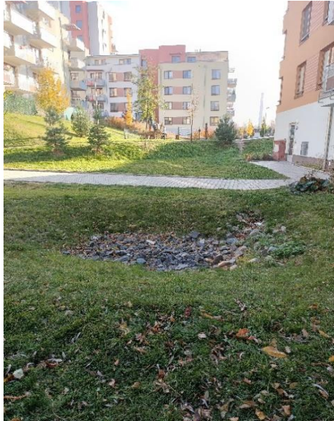
Picture 1: showing a land sag which allows for water infiltration and retention as well as slower water outfall into the recipient.
