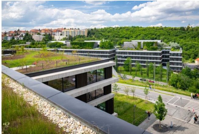
Picture 5: showing part of the ČSOB headquarters in Prague – Radlice Visible is a green roof as well as green permeable surfaces around the building (Nadace Partnerství b, 2022).
