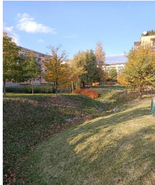
Picture 2: showing a land sag which allows for water infiltration and retention as well as slower water outfall into the recipient.
