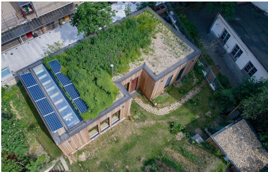
Picture 6: a bird's view on the roof of the house. Visible are solar panels as well as the wetland roof (Nadace Partnerství d, 2022).
