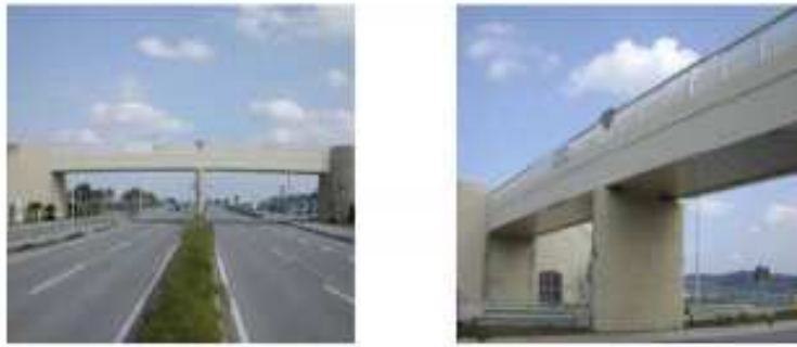
Figure 2.6: Pedestrian Bridge in Okinawa, Japan made of Hybrid Composite [76]
