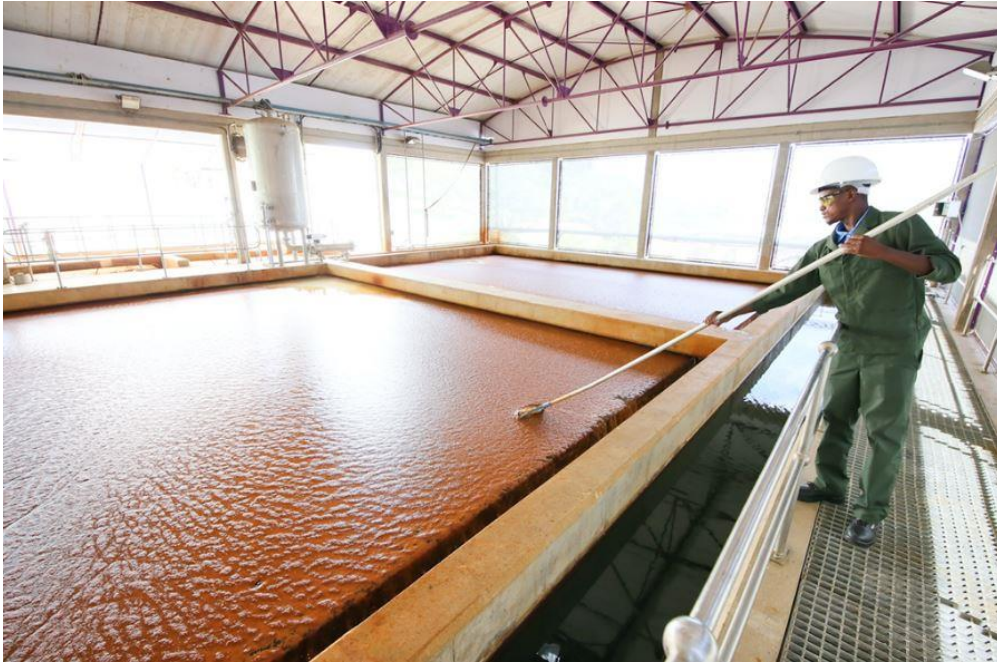
Figure 9: Employee inspecting effluent during the treatment process at the GWRP
