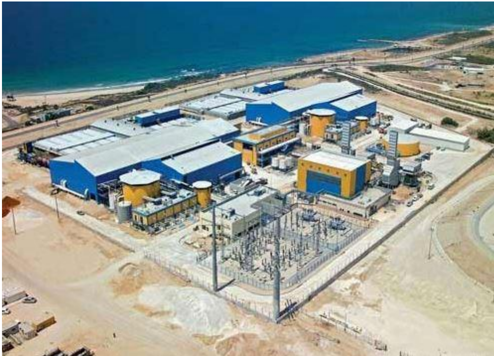
Figure 10: Ashkelon Seawater Reverse Osmosis Plant, Israel
