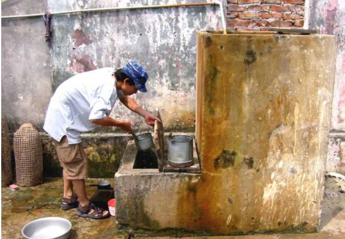
Figure 9 Sand Filtration Plant in North Vietnam
