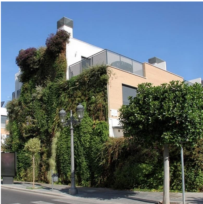
FOTO 34: Zelená fasáda ve Valencii, 2010 ( http://www.paisajismourbano.com/en/project-in-valencia-green-facade-in-paterna ).
