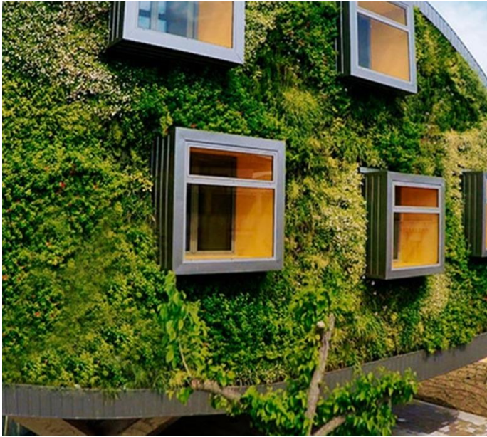
FOTO 33: Smart building, Malága, 2015 ( http://www.paisajismourbano.com/en/smart-green-building-in-alhaurin-de-la-torre-malaga ).
