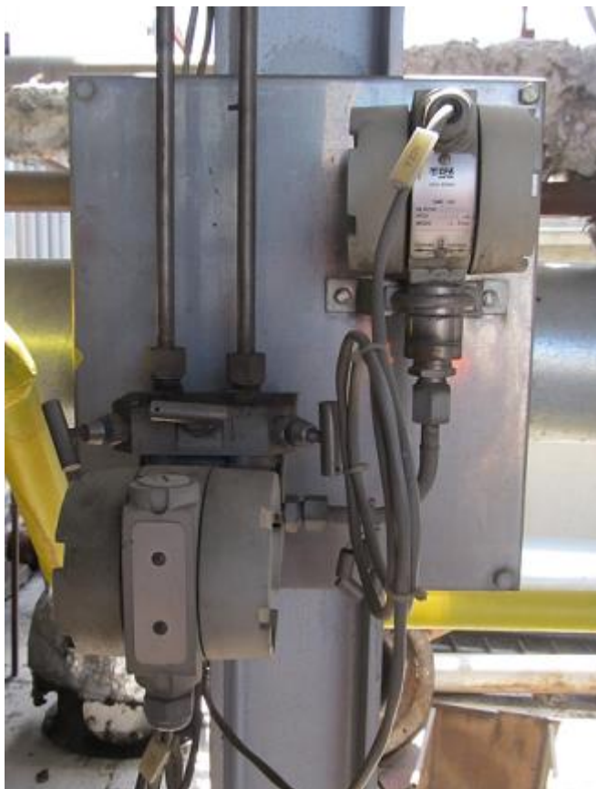
Figure 20 : Sensor of pressure loss in fluidized bed gasification reactor.
