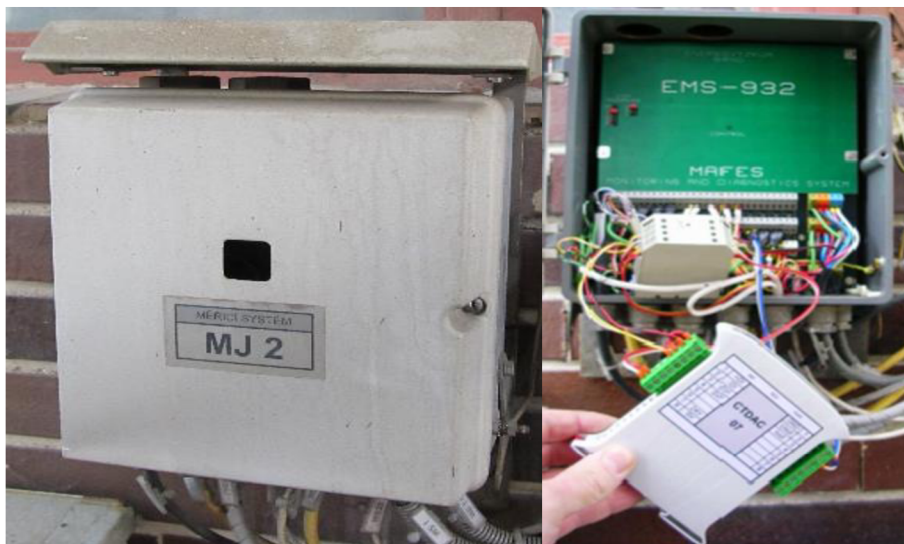
Figure 17: Measuring units MJ2 in laboratory (outdoor installation)
