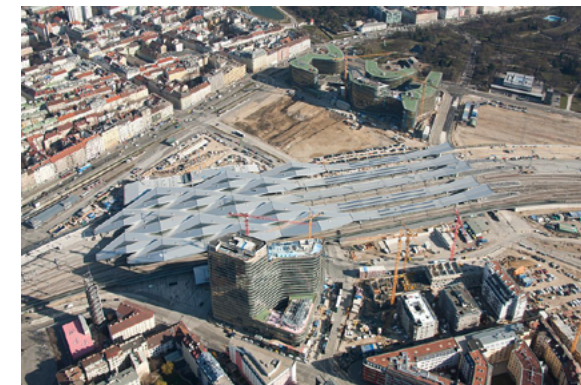
Figure 3: Newly created public transport hub provides a connection between the districts Favoriten and Wieden in Vienna, which were so far separated by the freight yard.
