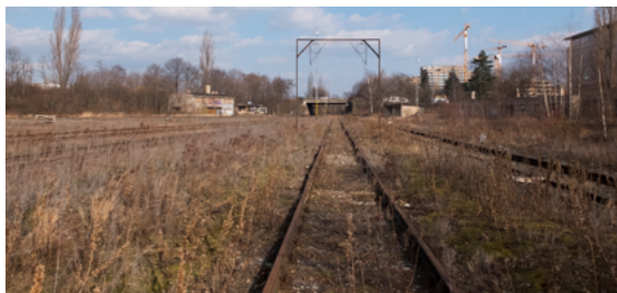
Figure 33: The very neglected part of the site in its eastern part - abandoned and ruined.
