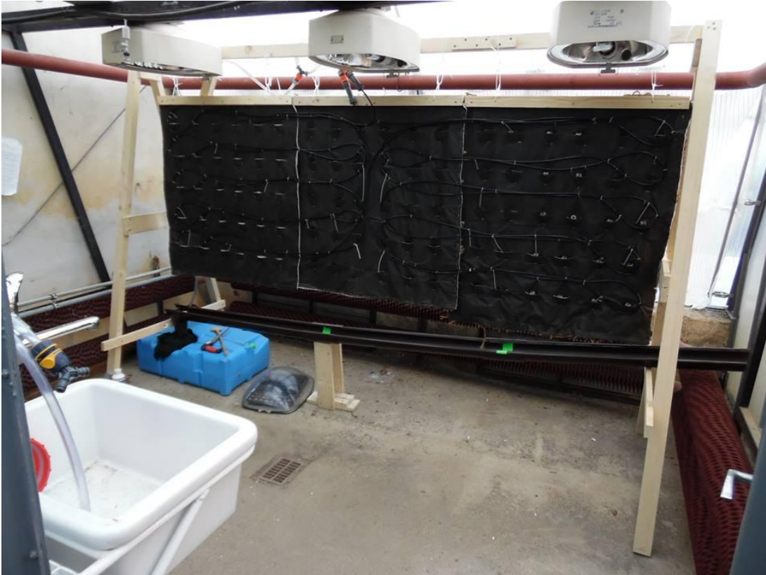
Figure 9: Complete constructed living wall system with framework and hydroponics irrigation system at the beginning of the germination phase (Photo: Author).
