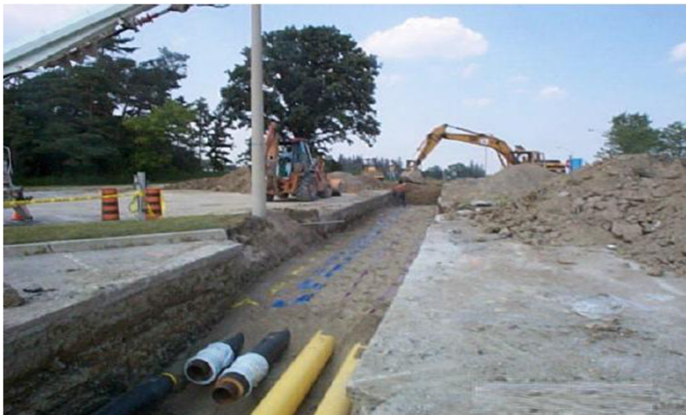
Fig. 10.2 Typical piping installations [32]
