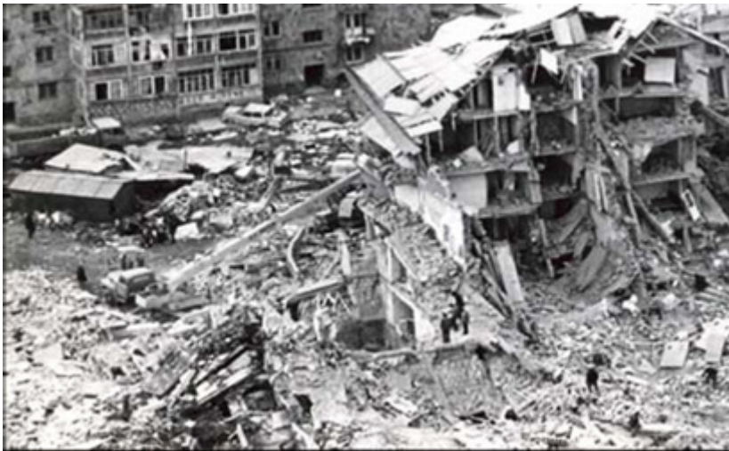
Figure 26: Residential building after disaster Source: newizv.ru
