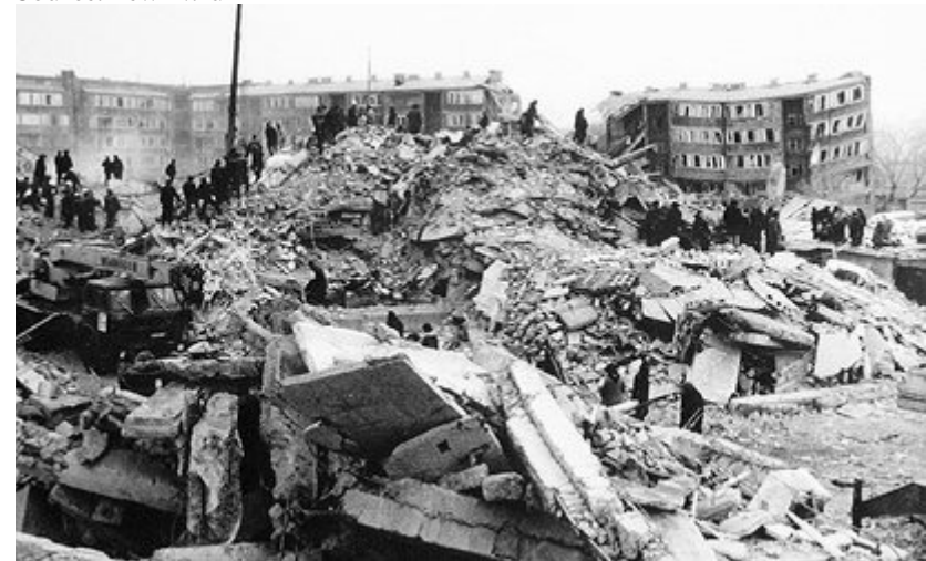
Figure 27: Residential building after disaster Source: newizv.ru
