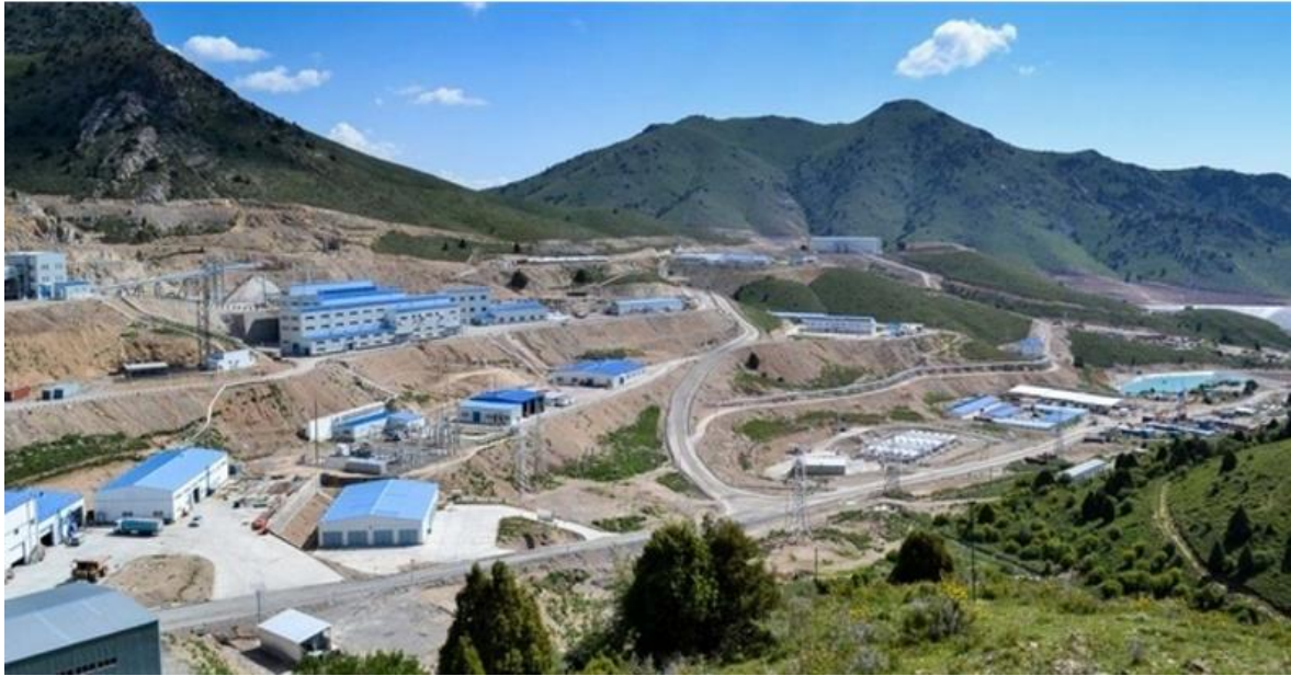
Picture 3: Bozymchak mine
