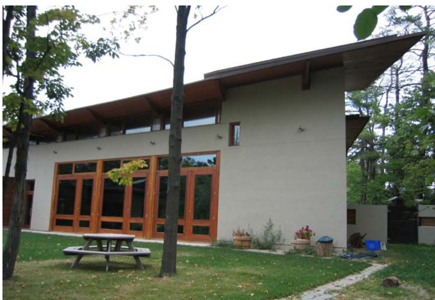
obr.8 Kostel v Oakville, Ontario, Kanada, autor Steven Teeple, 2007.
