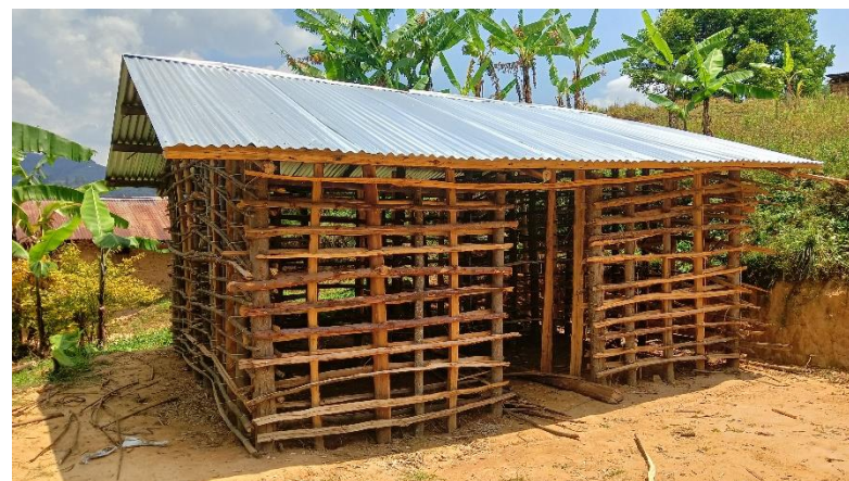
Appendix Figure 10: Mud house construction in Nyabaremura
