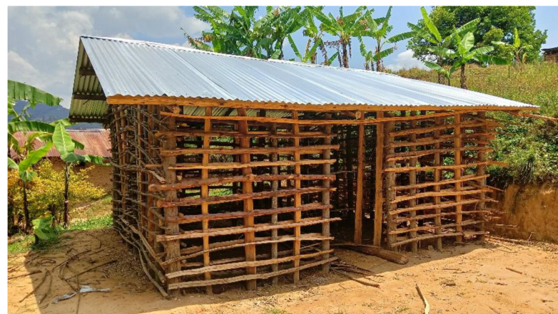
Appendix Figure 10: Mud house construction in Nyabaremura
