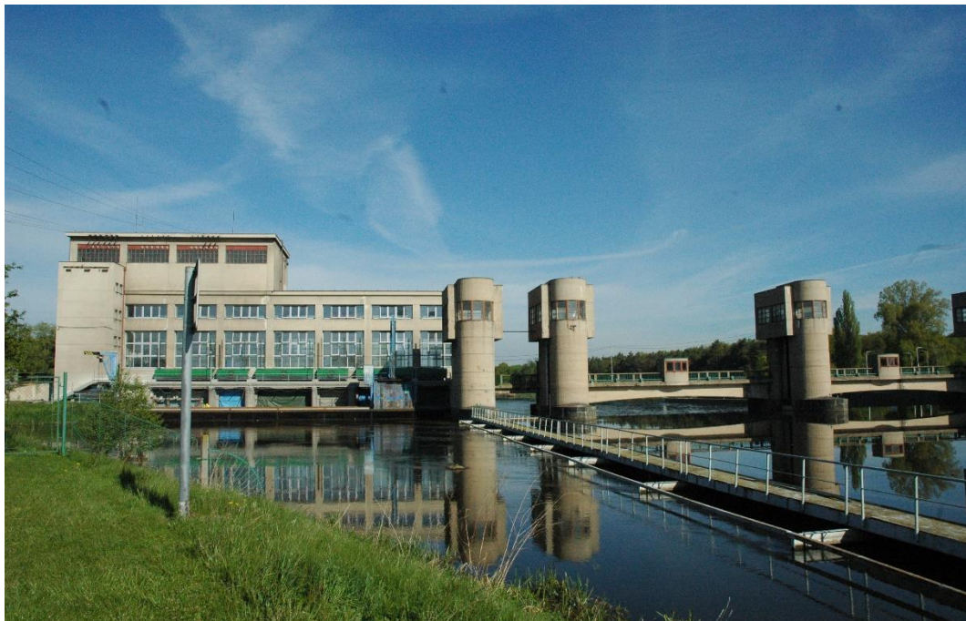
Obr.42 MVE Kostelec nad Labem
