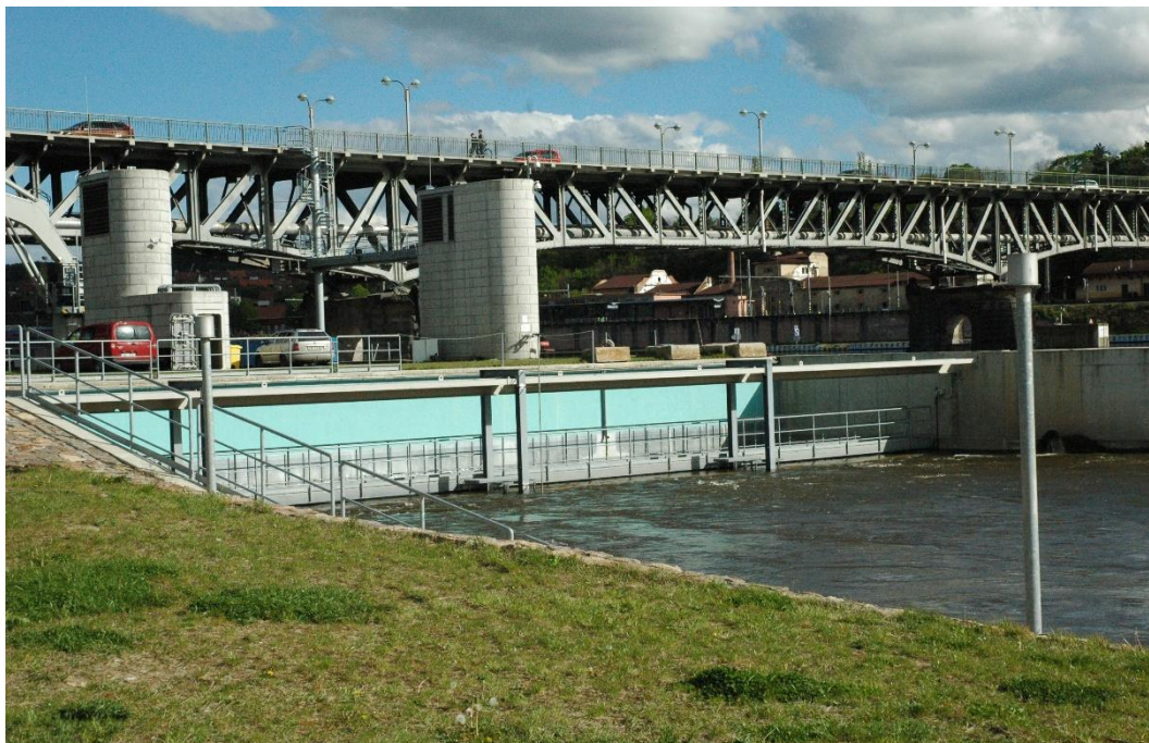
Obr.54 MVE Roudnice nad Labem
