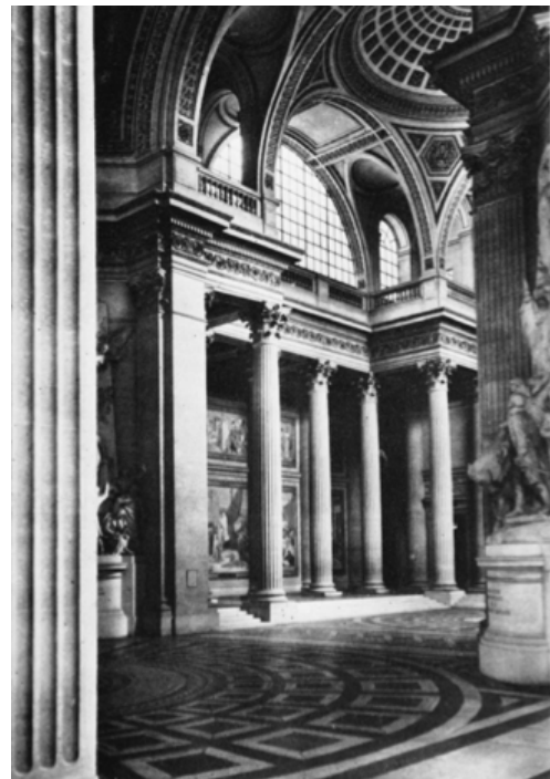
Figure 6: Corinthian columns inside the Saint-Geneviève church-Parisian Panthéon, in: Allan Braham, "Drawings for Soufflot's Sainte Geneviève," In: The Burlington Magazine , Vol. 113, No. 823, (Burlington Magazine Publications Ltd., 1971): 592.
