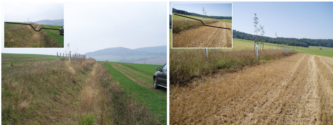
Figure 4 Newly built lynchets constructed within antierosion arrangements.
