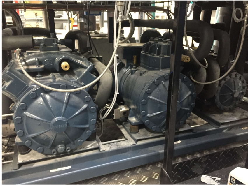
Figure 4.2 R744 piston-type compressors pack. Base-load compressor (Dorin CD1400H) at the left and parallel compressors (Dorin CD1000H and Dorin CD380H) at the right.
