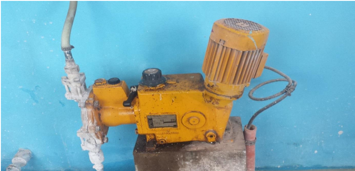
Figure 8: Device used to measure the quantity of \text{Ca}(\text{OH})_2 called “Doseuse”
