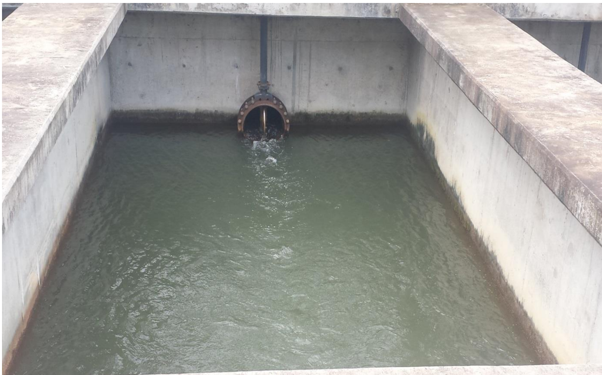
Figure 14: Rapid Filtration in the Yessoulou Plant
