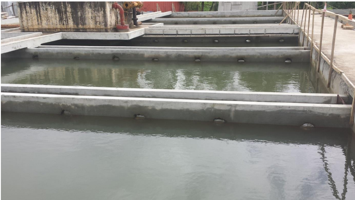
Figure 12: Settling (Decantation) process in Yessoulou
