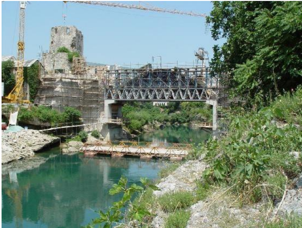
Figure 4.08 Old Bridge during the reconstruction, scaffolding. Mostar
