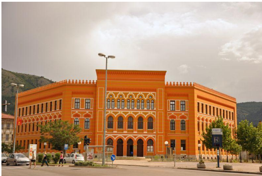
Figure 4.03 High School in Mostar after recovery
