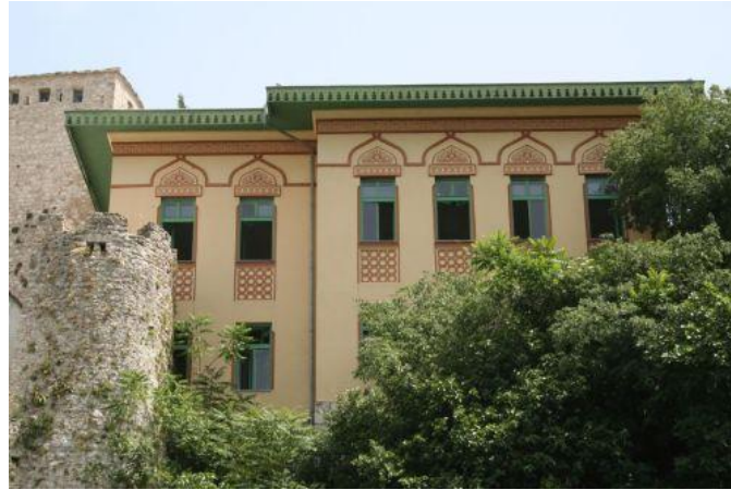
Figure 1.3 Ottoman house in Mostar
