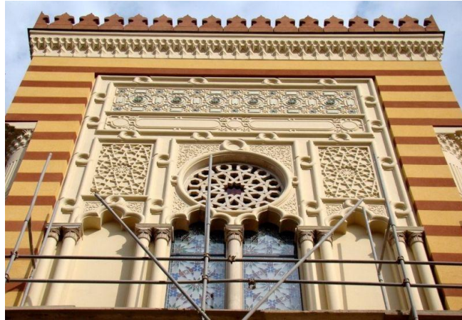
Figure 4.02 Detail during the façade recovery of Sarajevo Town Hall
