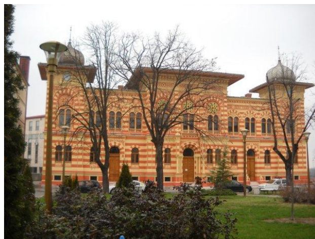
Figure 4.04 Town Hall of Brčko after recovery
