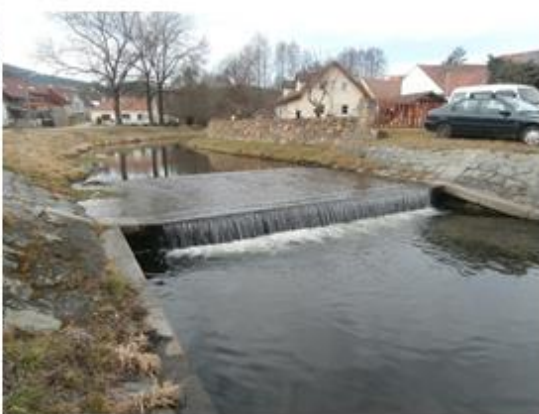
jez Novosedly ř.km 3.448
