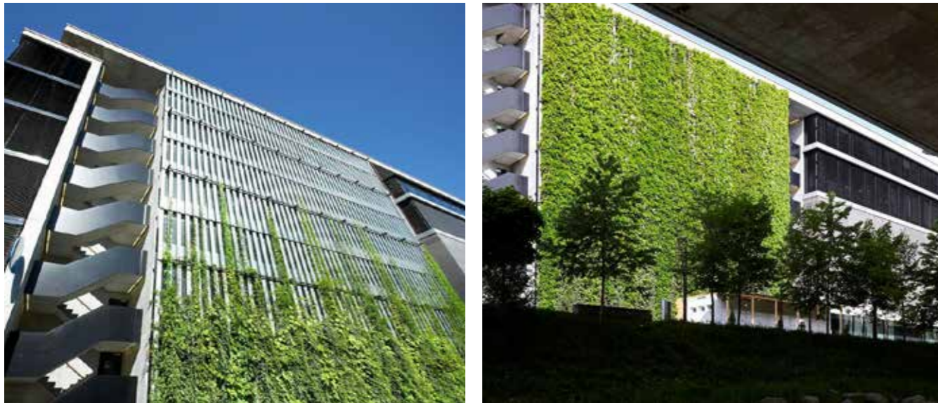
Obr. 18 a 19: Sihlcity Shopping centre Living facade (zdroj: Greenroofs 2007)
