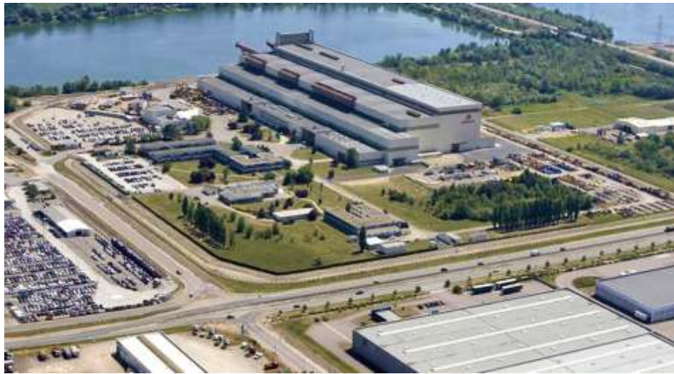
Fig. 2 Framatome Saint-Marcel plant [31].
