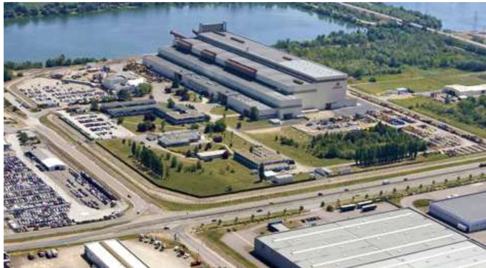
Fig. 2 Framatome Saint-Marcel plant [31].
