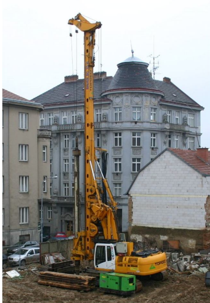
Obr. 24: Vrtná souprava BAUER BG 15 H
