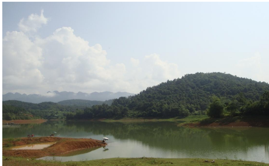
Picture 1: The water level was dropped during the irrigation season
