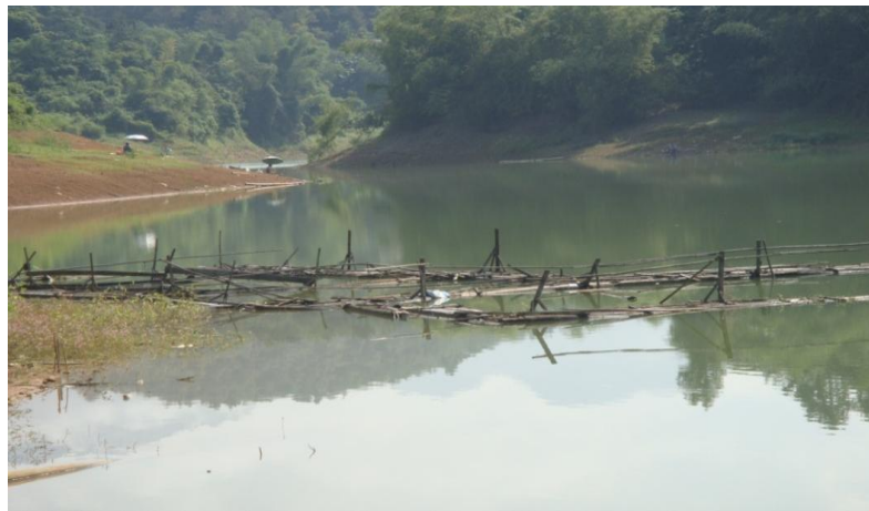
Picture 2: The damage of fish cages
