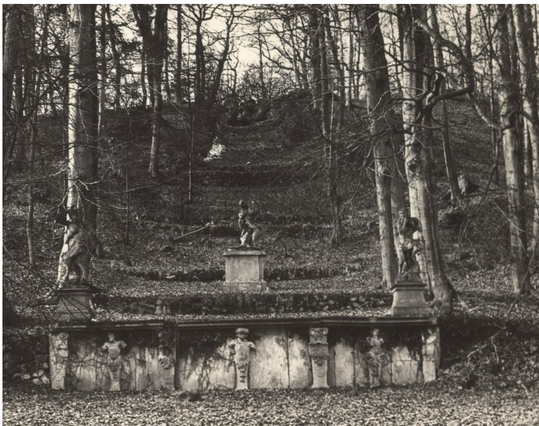
Figure 3.1.4 Archival photo of the cascade ruins with the large baroque fish at the top (The archives of Valeč 2013).
