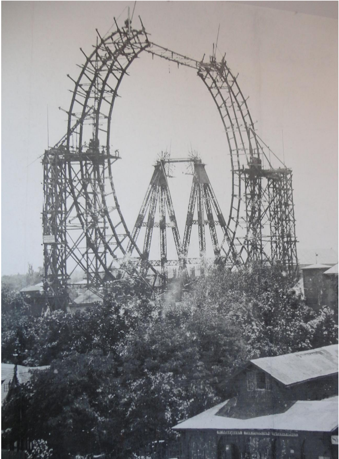
Figure 4: Historical photo of construction of Ferris Wheel in Prater Amusement Park. (Source: Author's archive)
