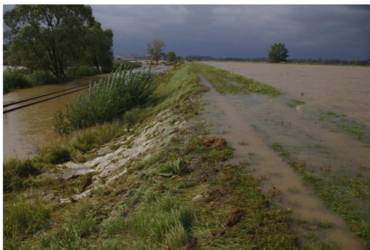
Fig. 6.5 Second phase: overtopping - no erosion
